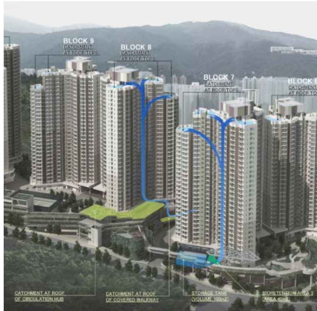
Source: AECOM, 2014. Mock-up of bio-retention Rainwater Harvesting System in Shui Chuen O Phase 1—Summary report for Hong Kong Housing Authority
