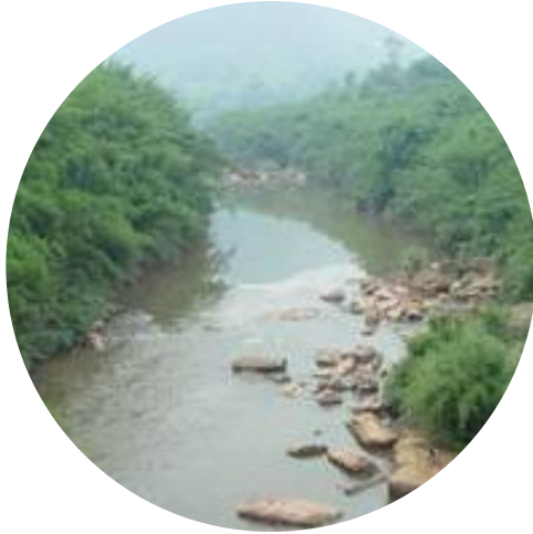
River bank stabilization
