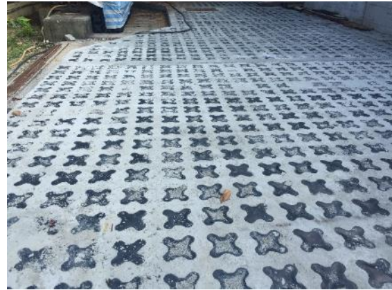
Figure 5: Grasscrete under Construction (2)
