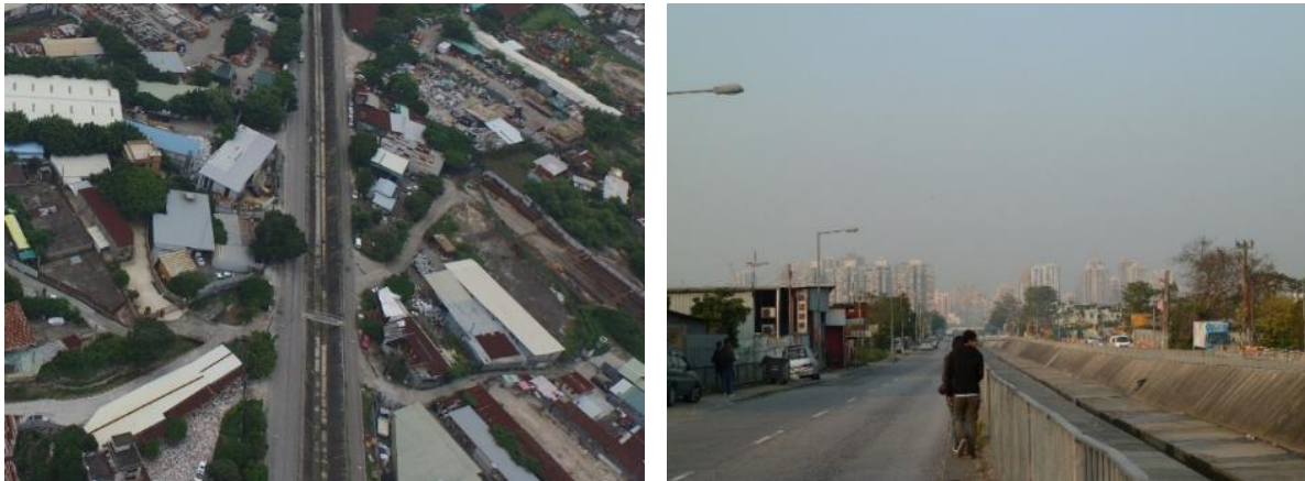
Figure 2: Photos of existing Yuen Long Nullah
