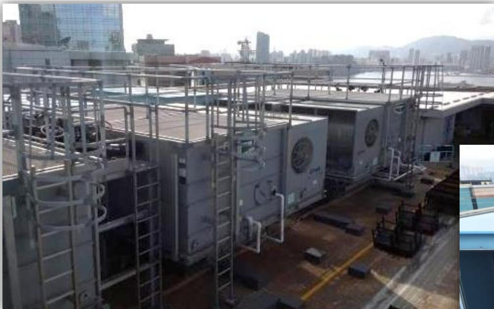
Cooling tower with variable speed condensing fans
