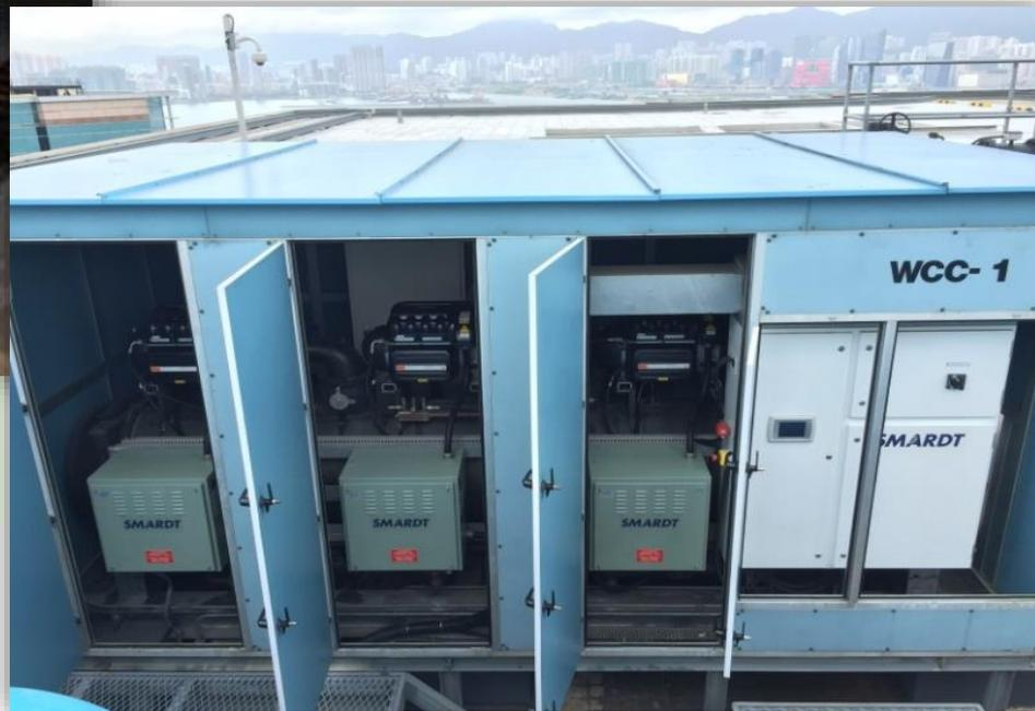
Enclosure for oil free centrifugal chiller
